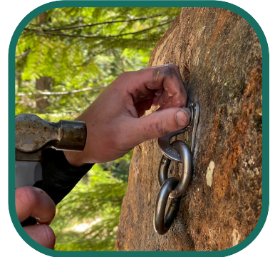
Above: Replacing hangers in Mineral Creek.
